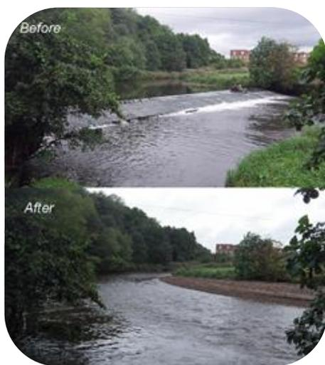
Barriers such as Goshan weir on the River Roch close to Bury (pictured) are being removed to reconnect sections of the river. Providing these connections allow the river to work more naturally improving silt and gravel movements and increasing the diversity of habitats available within the river. Fish and the insect life they feed on, together with otters, water voles and birds such as the kingfisher and the dipper all exploit these habitats.
